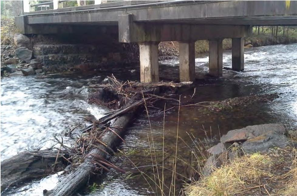
**Figure 4-5** Debris on the pier of the bridge on the Buxton-Marysville Road near No.562. Photo by Oxley & Partners, July 2014.
