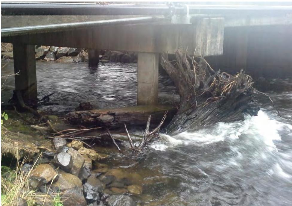
**Figure 4-4** Debris on the pier of the bridge on the Buxton-Marysville Road near No.760. Photo by Oxley & Partners, July 2014.
